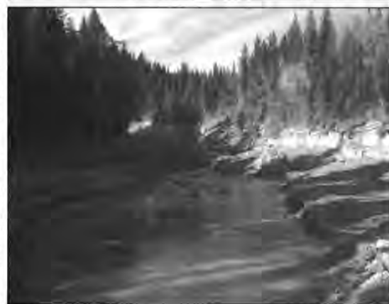
Hazeltine Creek in October 2008 before the mine disaster (top) and in October 2014, (above) after the dam breach. Photos courtesy Quesnel River Research Centre, University of Northern BC.
