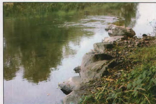
J Hooks face up-stream at a 30° angle.
