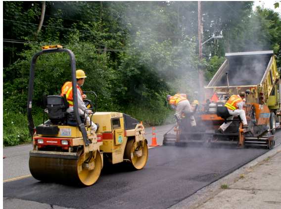
SR 7 Paving Project
