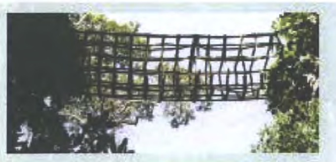
Figure 7.3 Canopy bridge installed near Lake Tinaroo, Australia, by Rupert Russell in 1995.
