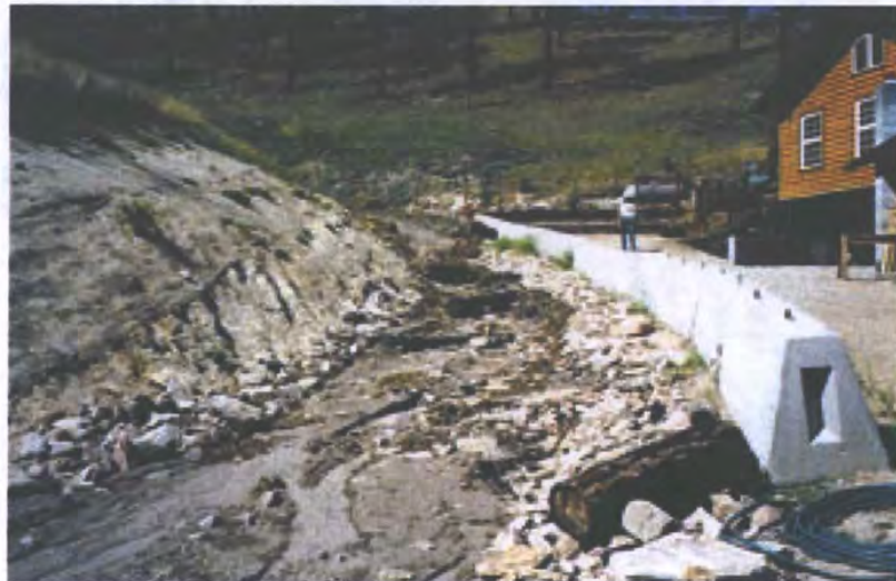
Figure C6. Example of creek channel lining using rock, Dickson Creek, Montana, USA. (Photograph and graphic, U.S. Department of Agriculture.)
