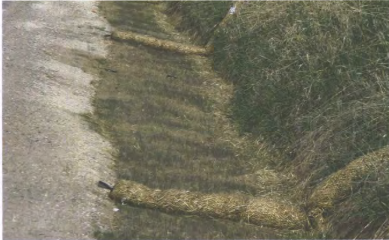
Figure C11. Straw wattles on the side of a road capture sediment and hold it onsite, enabling seeds to settle and germinate, aiding the revegetation process. (Photograph by Lynn Highland, U.S. Geological Survey.)
