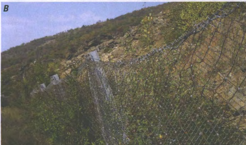
Figure C22. Protective rock barrier fencing along (A) a dirt trail in Pennsylvania, USA, and (B) a roadway in coastal California, USA. (Trail photograph, Lynn Highland, U.S. Geological Survey; roadway photograph from Federal Highway Administration, USA.)
