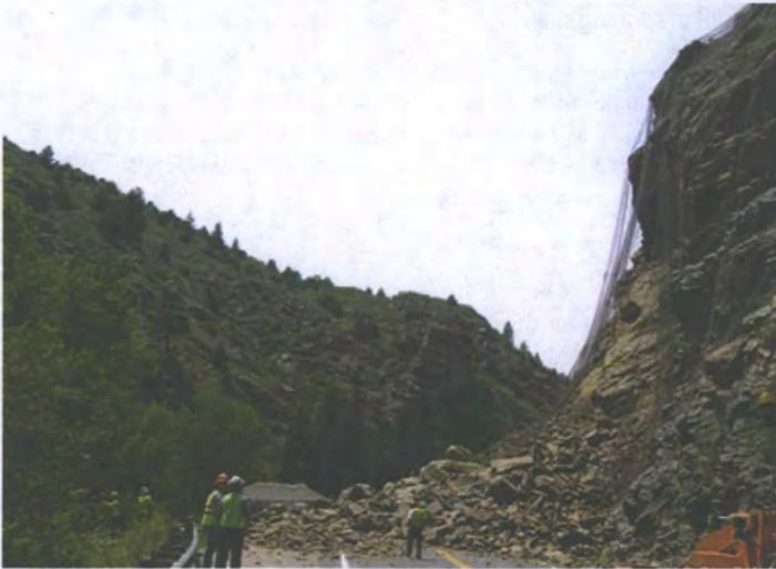
Figure 4. A rockfall/slide that occurred in Clear Creek Canyon, Colorado, USA, in 2005, closing the canyon to traffic for a number of weeks. The photograph also shows an example of a rock curtain, a barrier commonly applied over hazardous rock faces (right center of photograph). (Photograph by Colorado Geological Survey.)
