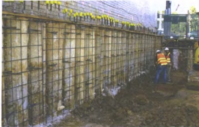
Figure C17. A concrete-filled pile wall. Reinforcing mesh has been hung over face of piles, ready for shotcrete spraying. Location is Brighton, Melbourne, Australia. (Photograph courtesy of Basement Construction Services, Victoria, Australia.)
