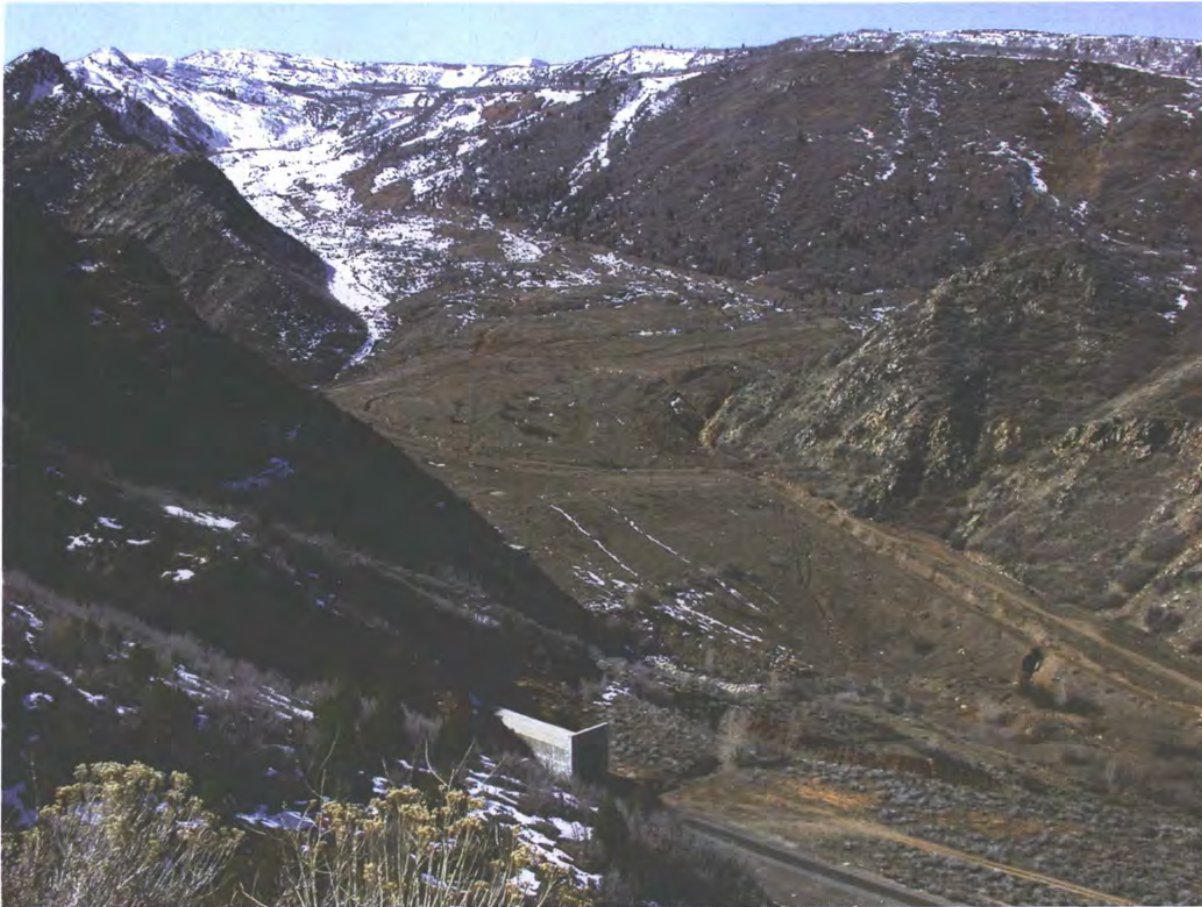
Figure 42. The Thistle landslide in Utah, USA. This 1983 landslide dammed the Spanish Fork River, backing up water that flooded the town of Thistle. Many landslide dams are much smaller than the one shown here and potentially can be overtopped by backed-up water, or eroded through. Some are much larger, and roads and railroad lines that are blocked or damaged must be diverted around the landslide mass. The concrete tunnel at the lower part of the bottom photograph shows where the rail line was rerouted around the Thistle slide and excavated through an adjacent mountain.
