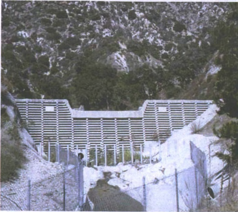
Figure C8. Upstream view of concrete crib-type check dam with low-flow center section in southern California, USA. (Photograph by Los Angeles County Flood Control District.)
