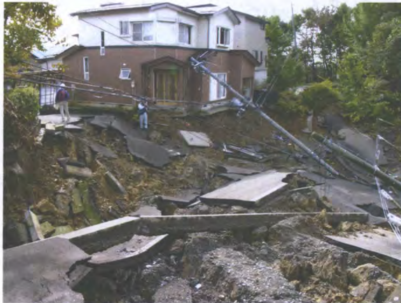
Figure 27. Earthquake-induced landslide damage to a house built on artificial fill, after the 2004 Niigata Prefecture earthquake in Japan. (Photograph by Professor Kamai, Kyoto University, Japan.)
