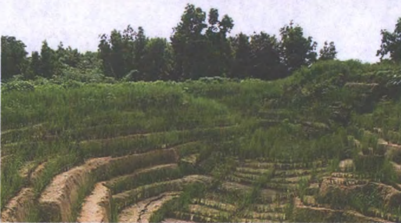
Figure C18. A Vetiver grass system is being used in the Democratic Republic of the Congo for gully control in urban areas and for highway stabilization. These gullies are a major problem in this area and other West African countries ( top ); the same slope now has improved drainage, and the slope has been planted in Vetiver grass ( middle ); this planting of Vetiver grass is about 3 months old ( bottom ).
