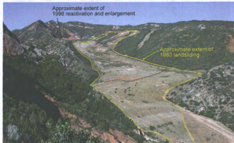
Figure C55. Photograph with annotations showing the reactivation and enlargement of the Thistle landslide dam. (Photograph courtesy of the Utah Geological Survey.)
