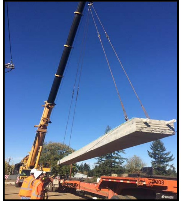
Fifth Plain Creek Bridge
