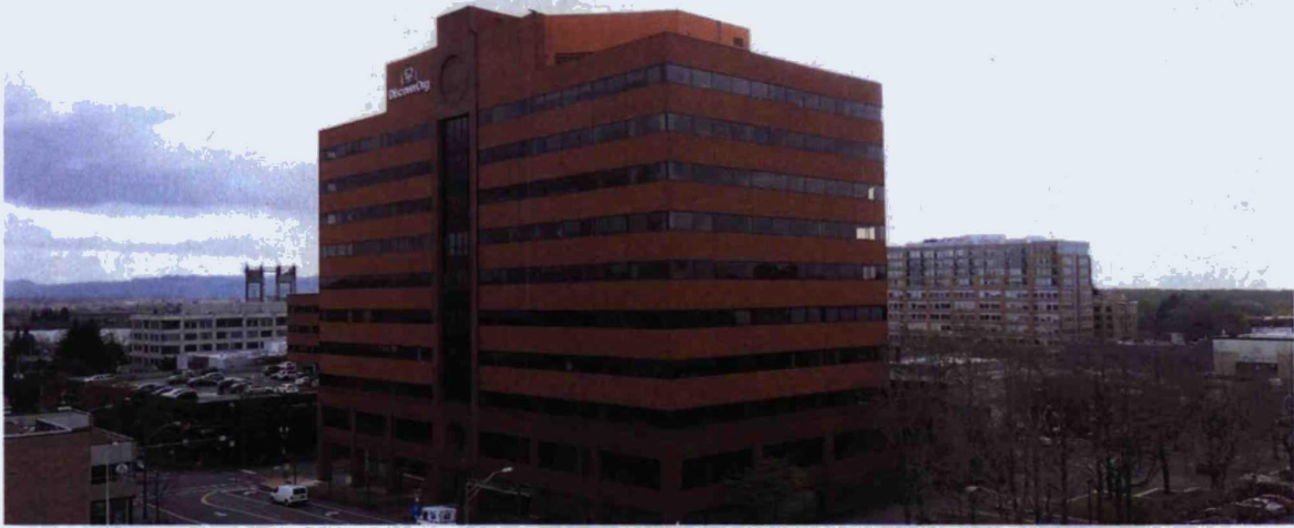
Looking south from C Street and Evergreen Blvd with Discover.org building closest to us, showing a handful of medium-sized high-rise constructions, a step in the right direction. 3-24-2016
